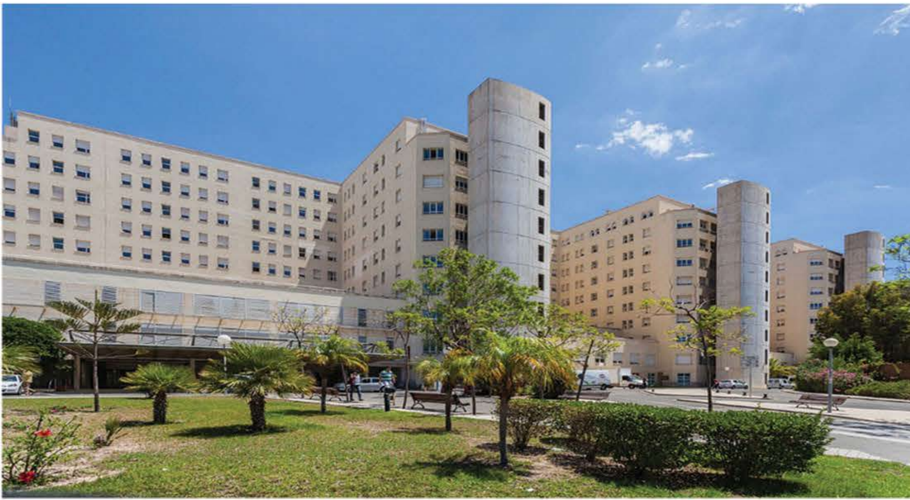
ALICANTE UNIVERSITY HOSPITAL | Alicante, Spain
