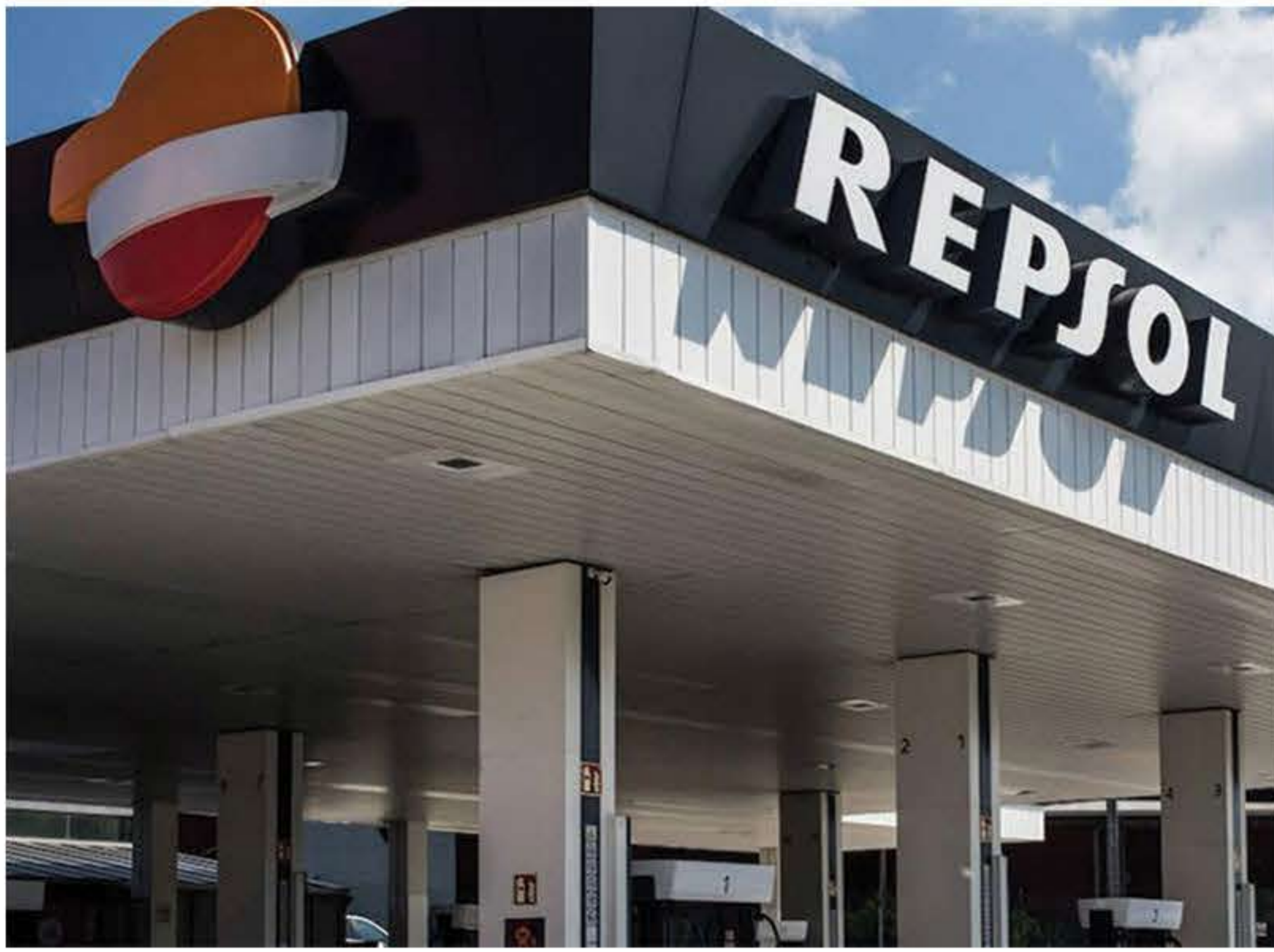
REPSOL REFINERY | Puertollano, Spain
